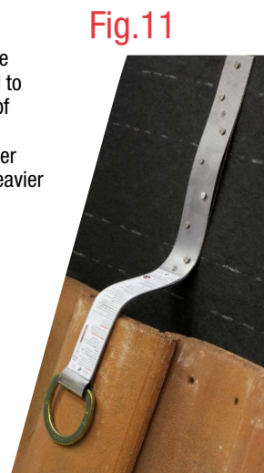
Conform Anchor Leg to the tile profile.
